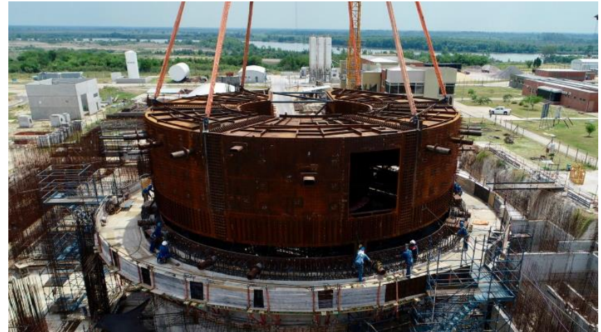
CAREM-25 Construction Site (Lima, Buenos Aires, Argentina) [2]
